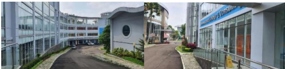
Figure 1 Front View of the Learning Building
