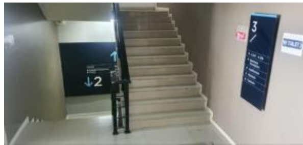
Figure 10 Learning Building Staircase Area
