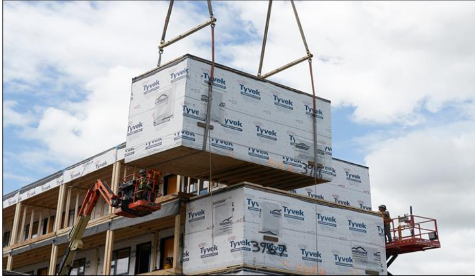
Figure 5 Modular Construction is Changing the Landscape and Building a Better Future. Accessed from https://www.nomodic.com/how-modular-construction-is-changing-the-landscape-and-building-a-better-future/
